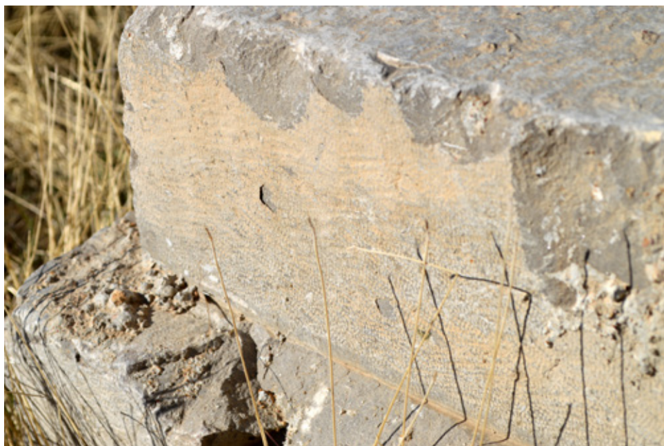
Fig. 6. Example of stone finished of Achaemenid toothed chisel marks on the column base (photo by author).
